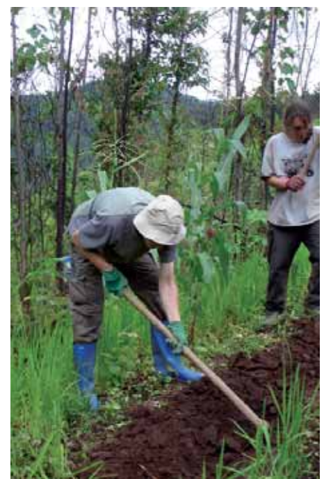
Thomas digging the pipeline
